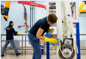
Step 1 First, the system is cleaned and disinfected
